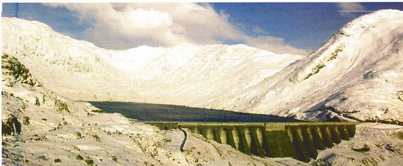
Cruachan power station: spot the cyber terrorist. Picture © Scottish Power.
